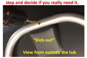
8.1: Make sure that your tub is centered within your frame and drill a hole above the two tub kick-outs (back and front of the cart) going through the pre-drilled holes in the aluminum frame. You would need a ¼" size drill bit and a powered drill.
